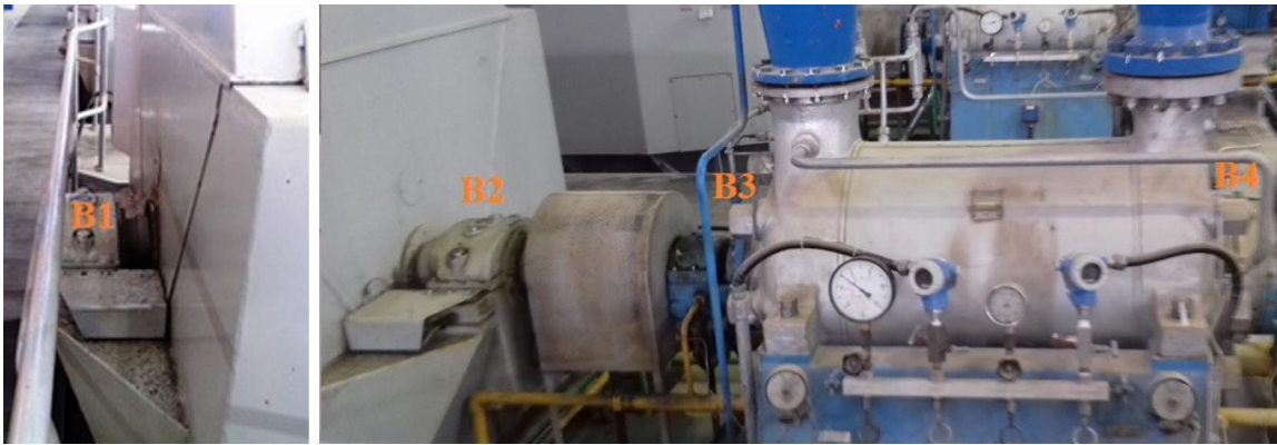
Figure 1. Pump Bearing Positions.
